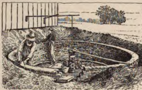
Fig. 70. Laying the foundation for a silo.
